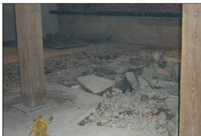
Basement Footings - April 2004
